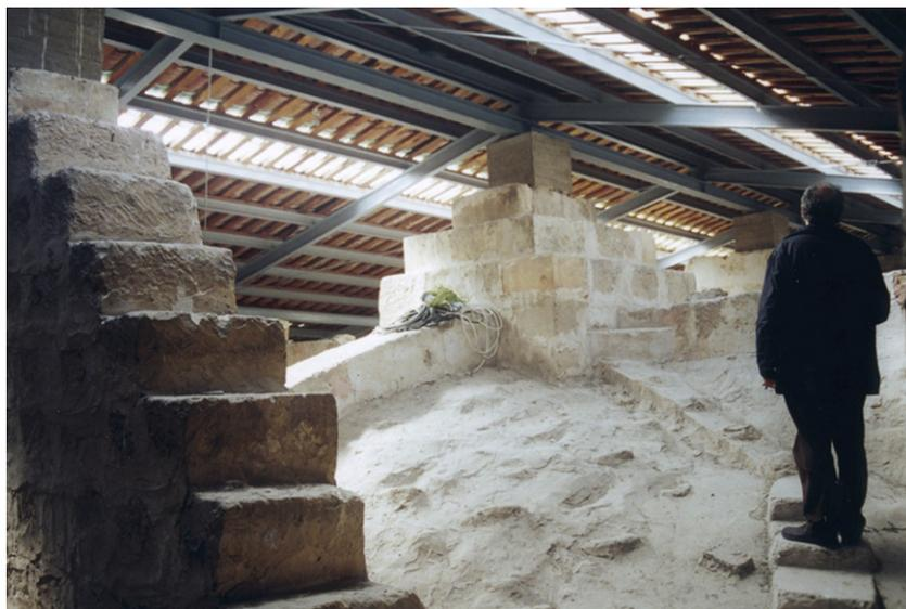
Fig. 3. Diaphragmatic arches with pyramidal dead weight over vaults.
